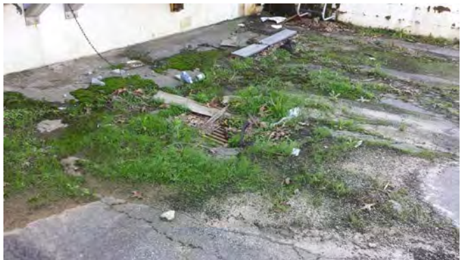
Drain Inlet at Loading Dock
