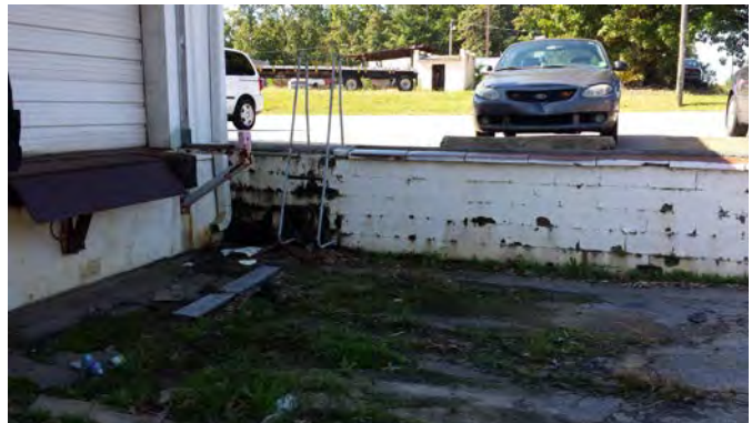
Retaining Wall at Loading Dock
