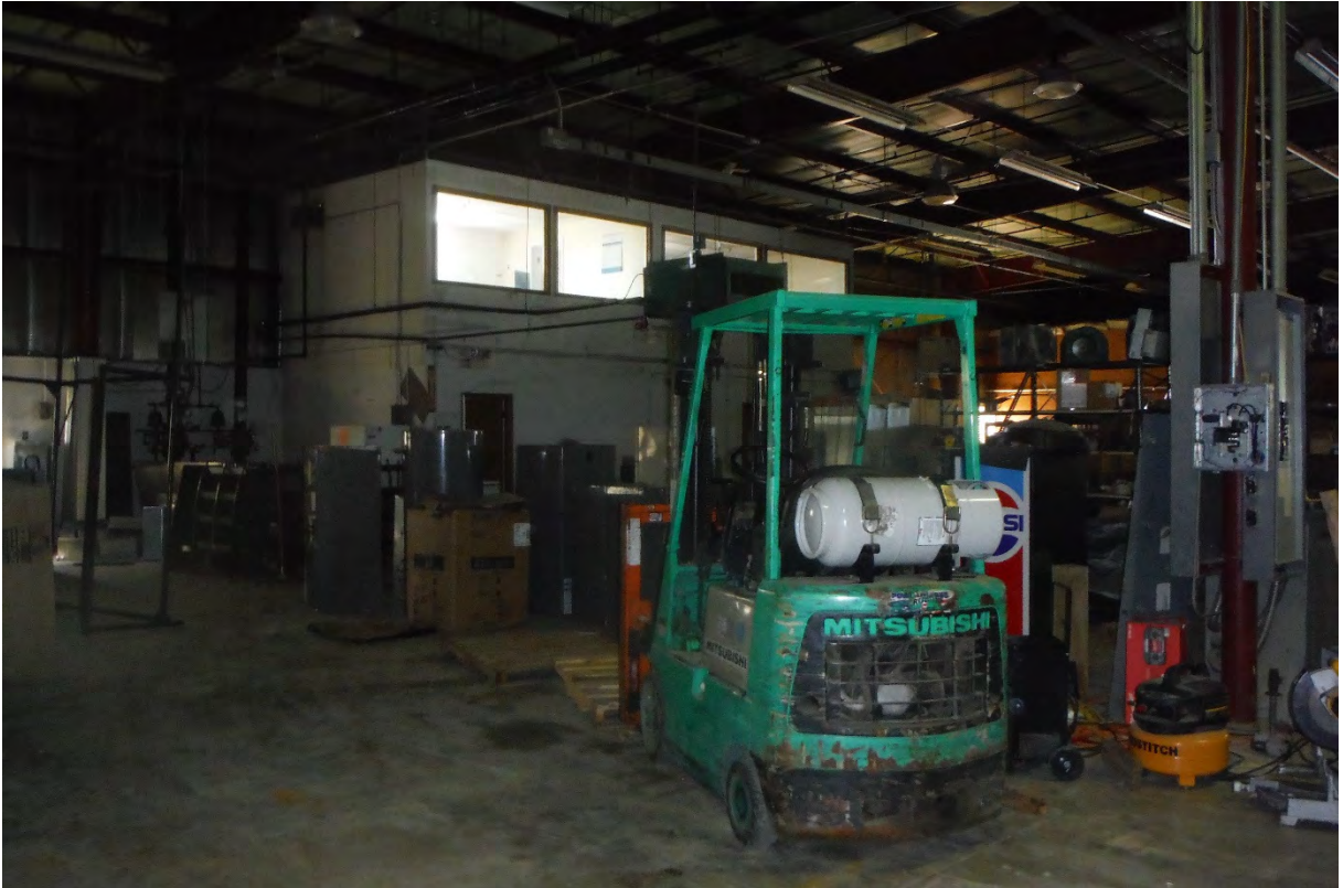
36. Photo taken of the southern wall of the southern warehouse. Second floor offices seen in center of frame. Minor superficial staining observed around the forklift.
