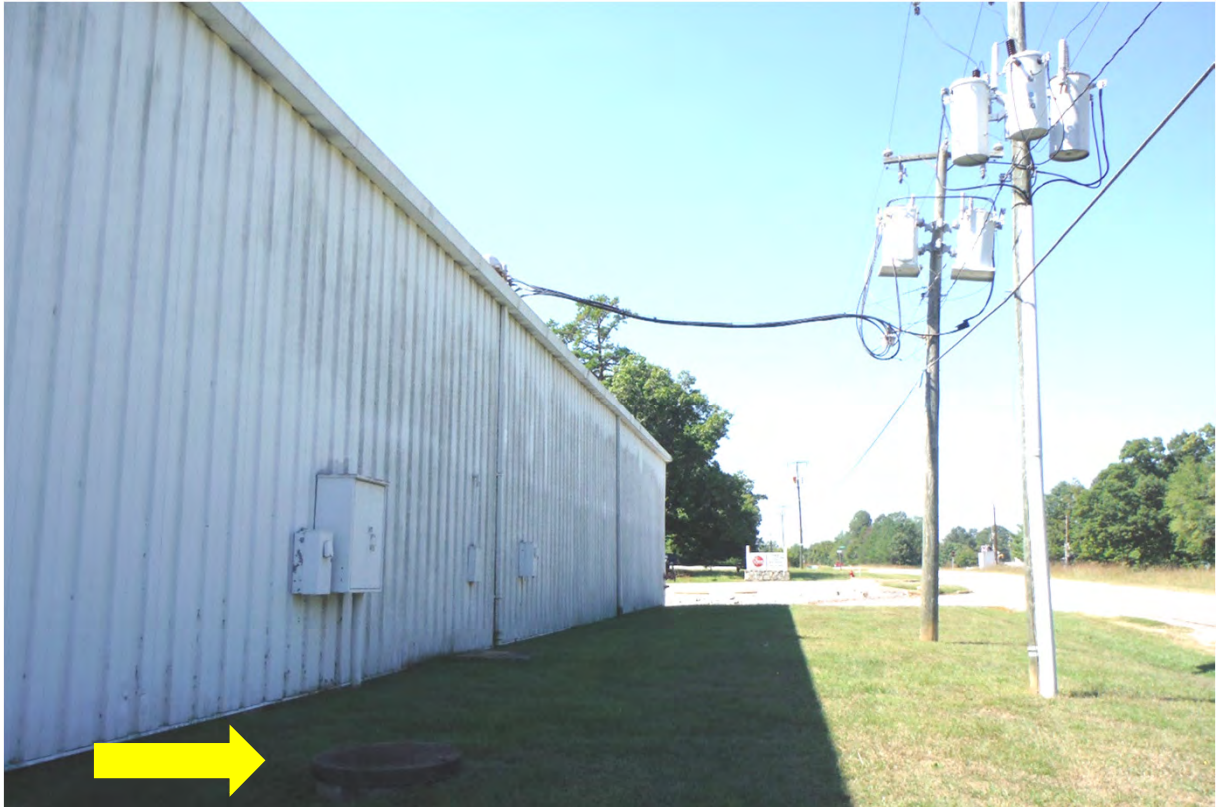
10. Overhead electric lines, electric boxes, and cement manhole riser (yellow arrow) observed on northern side of building.
