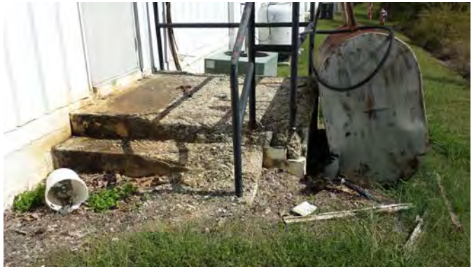
Existing Concrete Steps and Landing 1967 Metal Building
