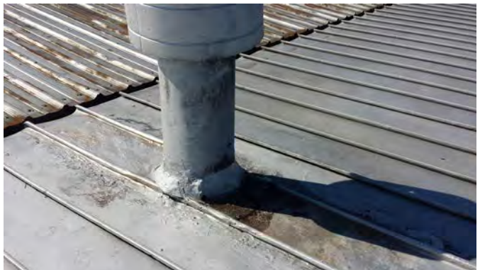
Typical Roof Penetration at Standing Seam Roof (1950 Metal Building)
