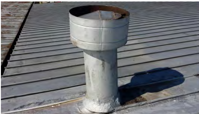
Typical Roof Penetration Over 1950 Metal Building
