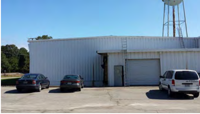
Exterior 1950 Metal Building, Loading Dock and Paving
