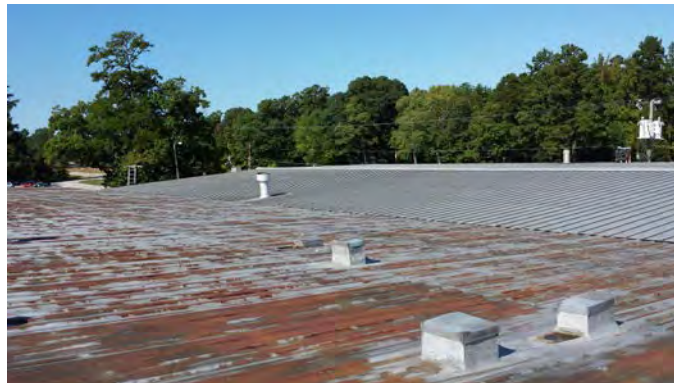
Overall View of 1950 and 1967 Metal Roofs
