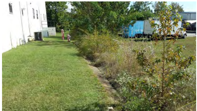
Concrete Drainage Swale at Rear of Property
