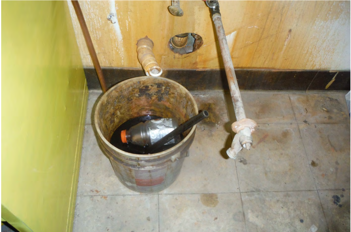
38. Uncovered bucket observed in petroleum/aerosol/paint storage area. No staining observed around the bucket.
