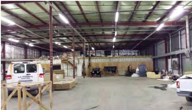
1950 Metal Building - Looking Towards Fitness Center
