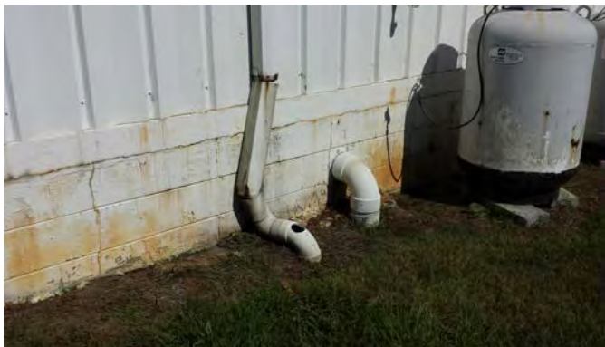
Foundation Wall and Downspout 1967 Metal Building
