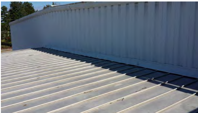
Metal Standing Seam Roof Over Lower Roof Adjacent to 1950 Metal Building
