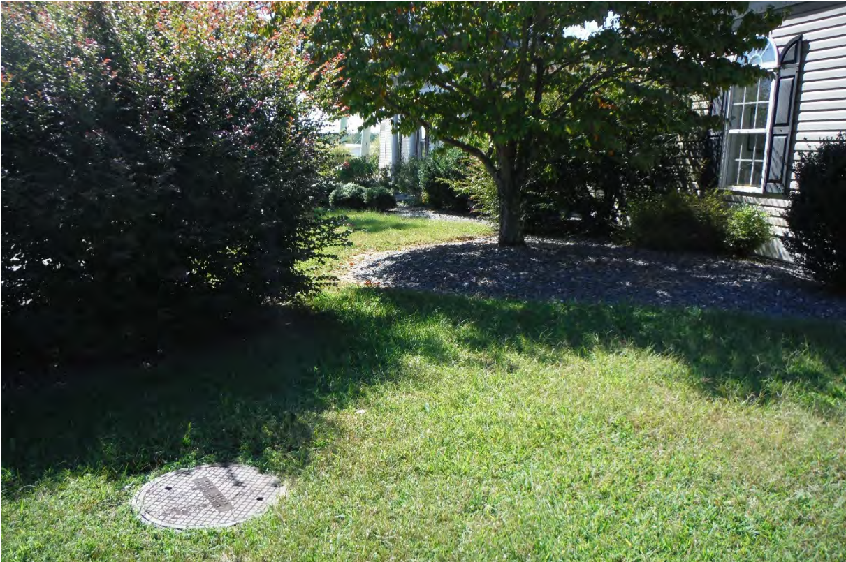
8. Water manhole cover observed near northeastern corner of building.
