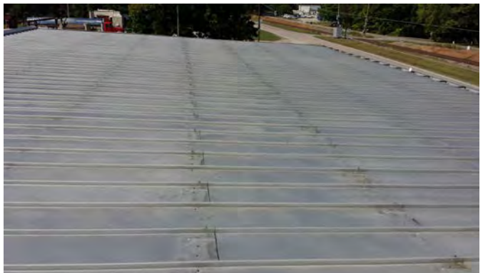
Standing Seam Roof Panels Showing Extent of Panel Laps (1950 Metal Building)
