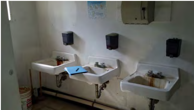
Typical Condition of Restrooms 1967 Metal Building (Borum Shop)
