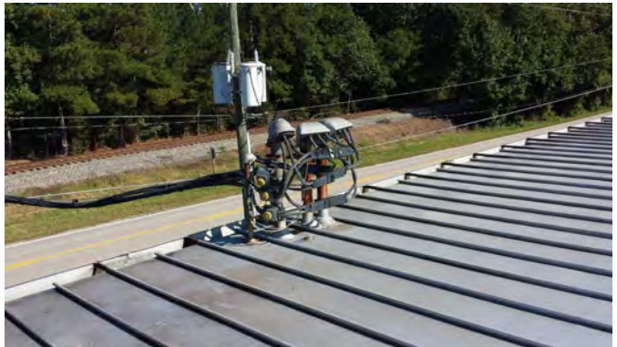
Weatherheads on 1950 Metal Building
