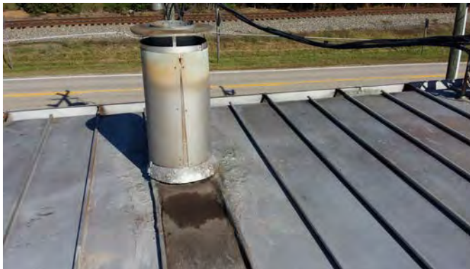
Standing Seam Roof and Flume at 1950 Metal Building
