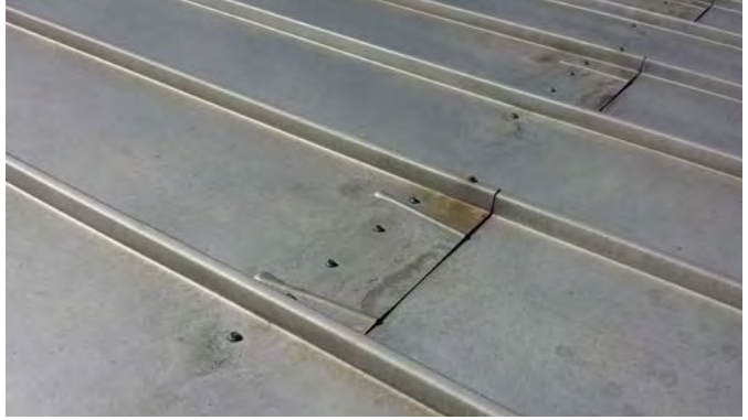
Typical Standing Seam Roof at 1950 Metal Building
