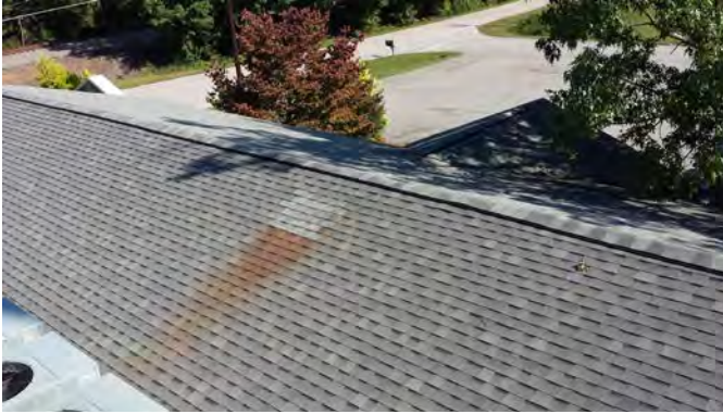
Shingle Roof Over Office/Fitness Center Area
