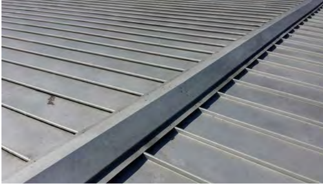
Non-Vented Ridge at 1950 Metal Building
