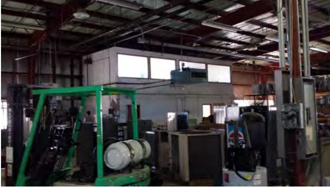
1967 Metal Building (Borum) Upper Office Area
