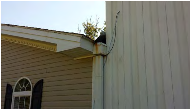
Downspout Draining Shingle Roof at 1950 Metal Building
