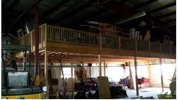
Elevated Storage Area - 1967 Metal Building (Borum Shop)
