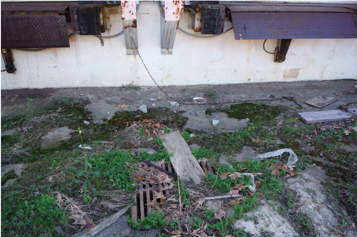
12. Stormwater drain below loading docks.
