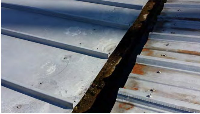
Gutter Between 1950 and 1967 Metal Buildings
