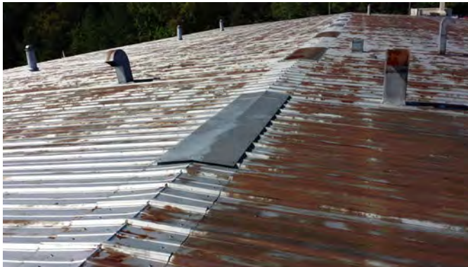
Ridge Repairs on the 1967 Metal Building (Borum Shop)
