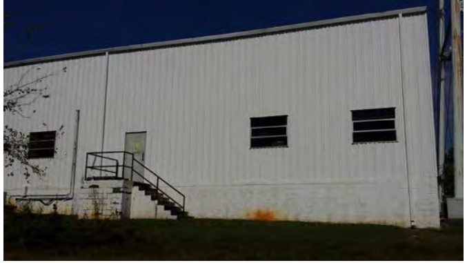
Existing Painted Block Foundation and Steps/Landing at 1967 Metal Building
