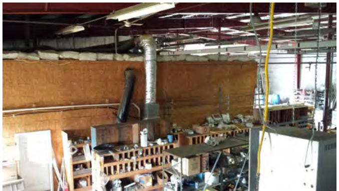
1967 Metal Building (Borum Shop) Towards Duct Fabrication
