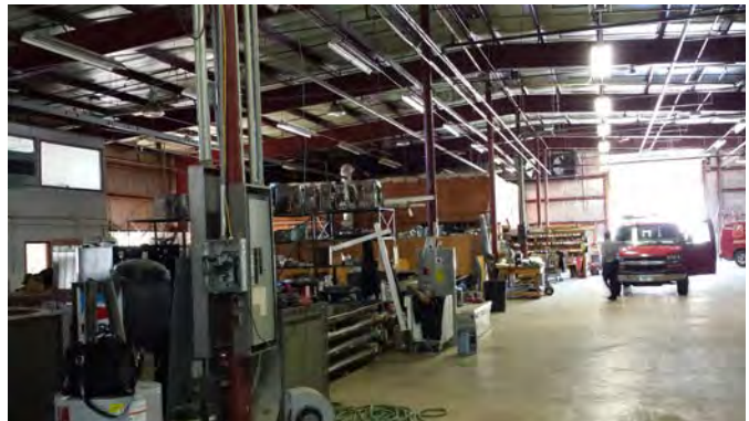
1967 Metal Building (Borum Shop)
