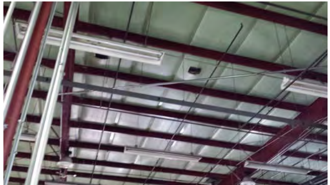
1967 Metal Building (Borum Shop)
