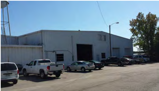
Exterior 1967 Metal Building (Borum Shop) and Paving
