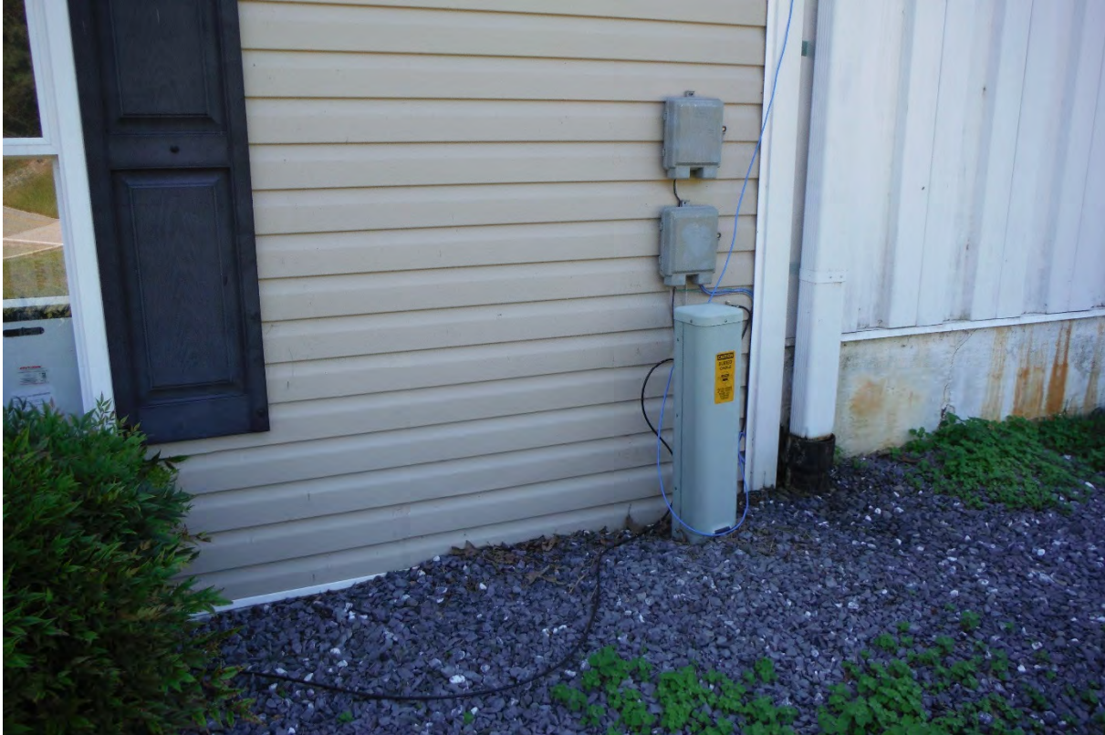
9. Telephone box and cables observed on northern side of building.
