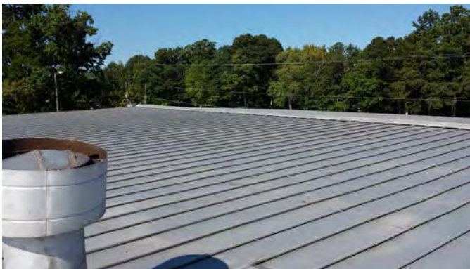
Typical Condition of Standing Seam Roof Over 1950 Metal Building
