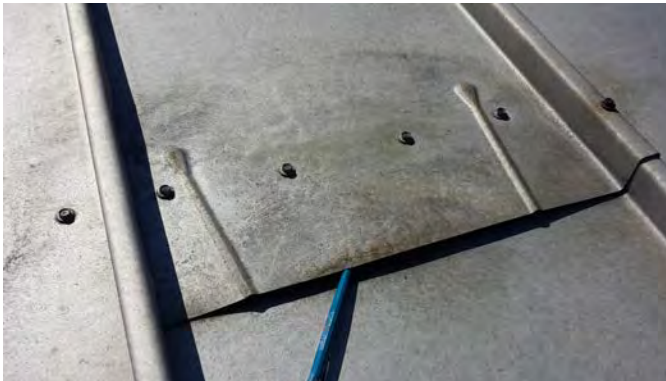
Typical Roof Panel Lap at 1950 Metal Building
