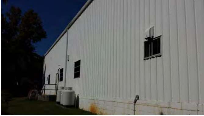
Foundation and Metal Wall Panels at 1967 Metal Building
